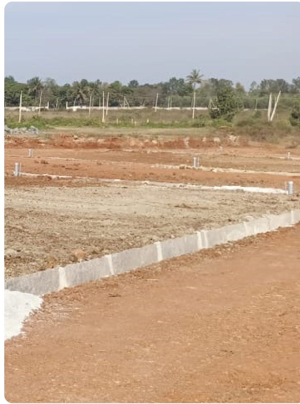
Work on Progress
